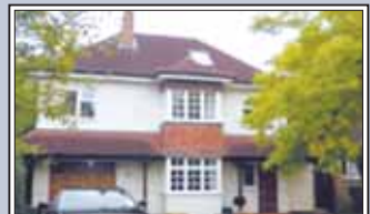
Old Oxted £2200 pcm A well presented 5 bedroom detached house. Set over three floors. Spacious living room. Fully fitted and newly installed kitchen. Master bedroom with ensuite bathroom.
